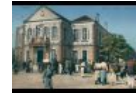
Dar al-Baladiyya, Damascus City Hall at the new urban centre at Merje Square 1900 Museum of Islamic Art at the Pergamon Museum, State Museums Berlin, Germany
