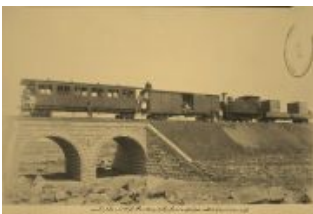
The Railway Bridge from Anatolia
